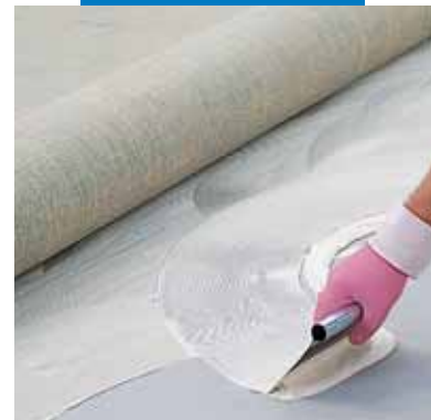
Installing linoleum with Aquacol T
