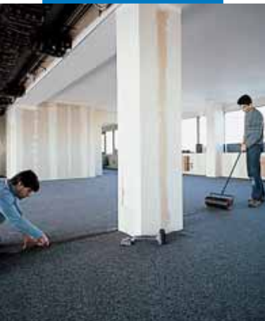
Pressing carpet joint with roller
