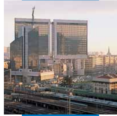
Corte Lambruschini, Genoa - 10,000 sq. metres of carpet installed with Aquacol T
