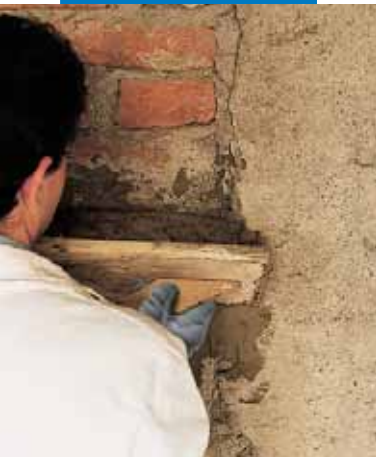
Restoring old brickwork
