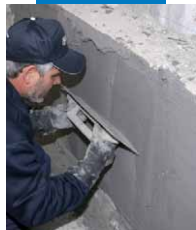
Application of Nivoplan with a float
