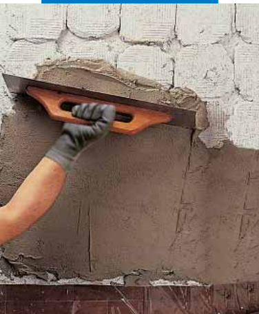
Levelling with a laying-on trowel
