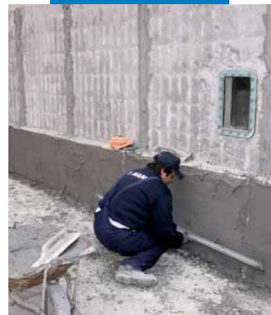
Levelling off the render with a straight-edge
